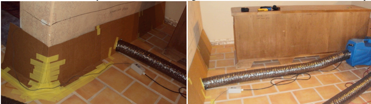
Leaning cardboard against the wall allows you to pump hot air in and "Focus" heats the wall.
